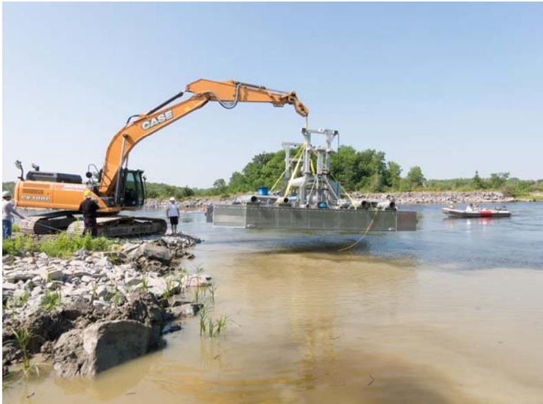
*Figure 4. The turbine being lowered into the river current*
